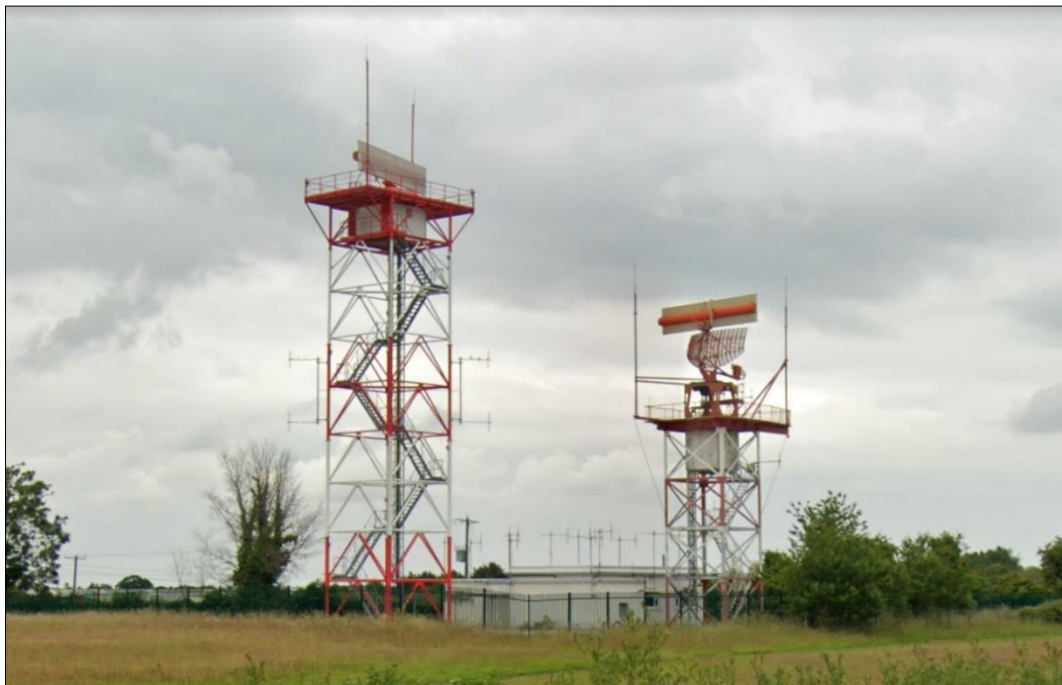
Figure 10. Dublin Airport MSSR Radar Station #2
